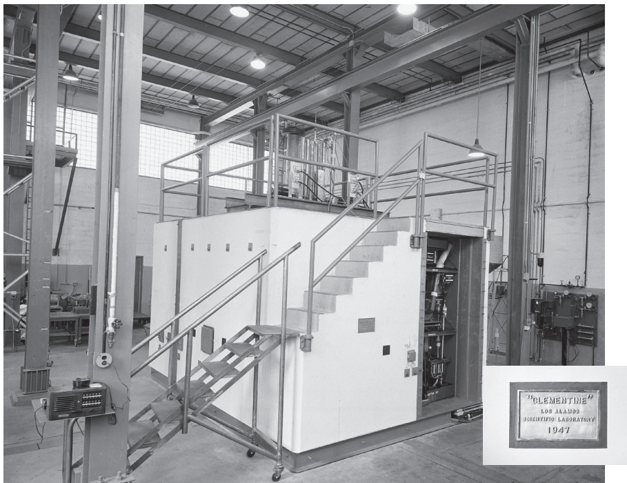
Figure 3. Complete structure of the Clementine reactor with stair access to the pile. Inset: Commemorative plaque on the stairs leading to the pile.
